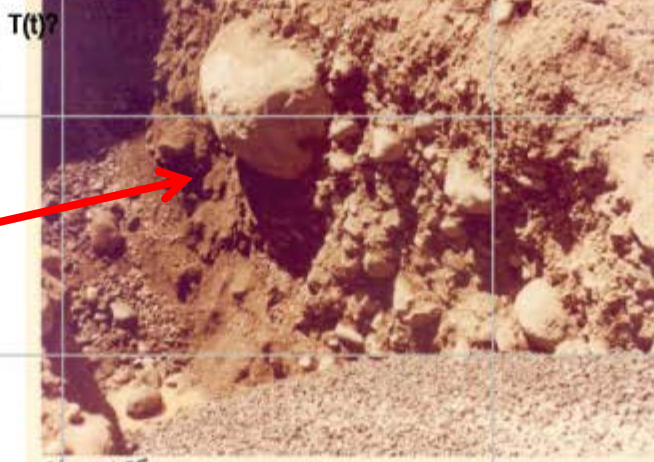
PHOTO 2. 1977 TOE DRAIN CONSTRUCTION AT STATION 2+75, 30' UPSLOPE FROM COLLECTION BOX SHOWN IN PHOTO 1 (OR OUT OF PHOTO 1). NOTICE LARGE BOULDER IN SIDE TRENCH MATERIAL AND "SUBDRAIN FILTER MATERIAL" (NO. 4 TO 1" AGG.) IN FRONT OF PHOTO.
