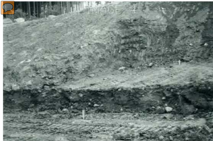
IMAGE 4: A VIEW OF THE RIGHT ABUTMENT IN AUGUST 1961. NOTE THE STEP IN THE GLACIAL TILL MATERIAL.
