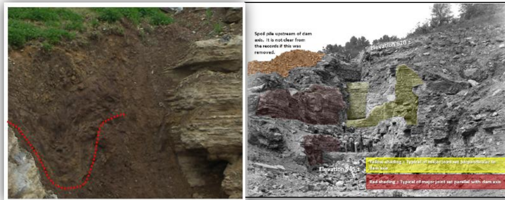
Figure 5. Left: Migration of soil into a karst feature at the left rim area of Center Hill dam. Right: Joint faces exposed in the core trench during construction of Center Hill Dam. quantified.
