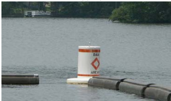
Buoy provides warning and the barrier system limits access
