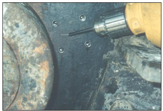
Photograph No. 8.—The 3/16-inch extra length drill bit position for drilling to trunnion pin.
