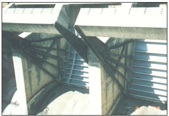
Photograph No. 2.—Back side of radial gates and gate arms.
