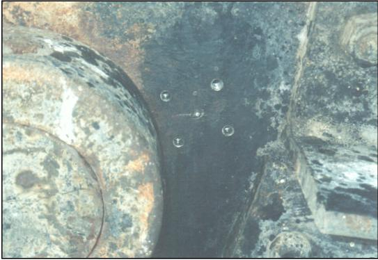
Photograph No. 7.—Grease block fitting mounting and grease channel hole placement on radial gate arm.
