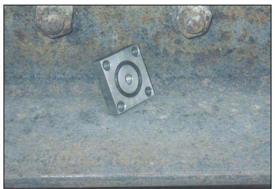
Photograph No. 6.—Grease block fitting with "O" ring installed.
