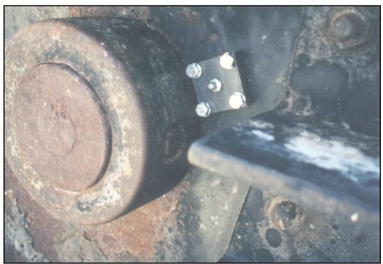
Photograph No. 9.—Installed grease block fitting on radial gate arm.
