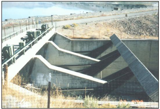
Photograph No. 1.—Radial gates as installed on the right embankment.
