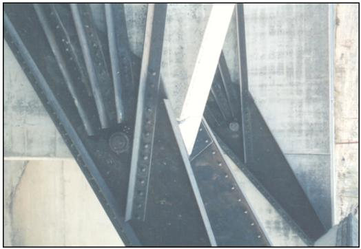
Photograph No. 3.—Spillway radial gate arms and pivot points.
