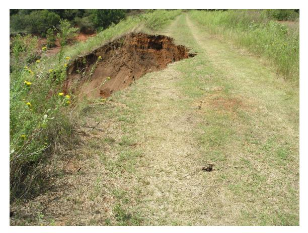
By mid-afternoon, the engineers had evaluated the situation as critical. Large cracks are found along the crest of the dam which indicated more sloughing is eminent. Minor sloughing continues. It is determined that the site is too unstable to try dumping rock into the void to help stabilize it. The next alternative is to get the water out as quickly as possible. The engineers on-site (the Project Engineer and the Resource
