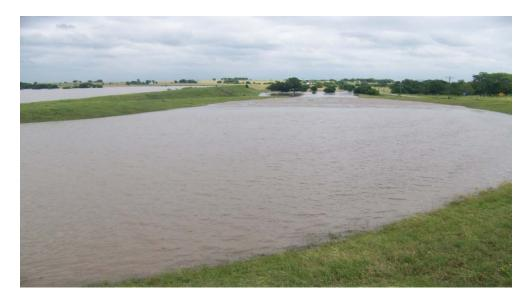
Figure 6: Auxiliary spillway functioning as designed
