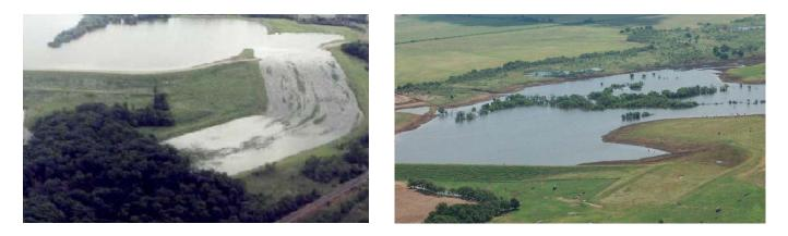
Figure 5: Auxiliary spillways are typically vegetated channels that safely convey runoff from large storms around the dam to avoid overtopping of the embankment
