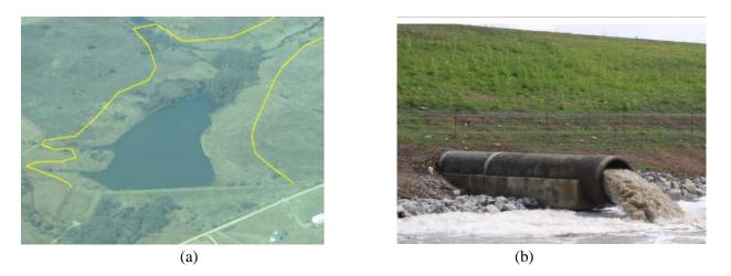
Figure 4: (a) Runoff from large storms is temporarily stored in the detention pool (below yellow line) and (b) slowly released through the principal spillway conduit
