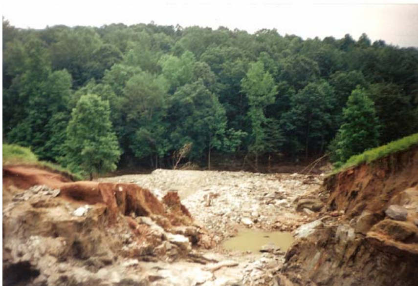
Figure 14: Damage to White Oak Dam emergency spillway, June 1995 (Photo courtesy of Rapidan Service Authority).
