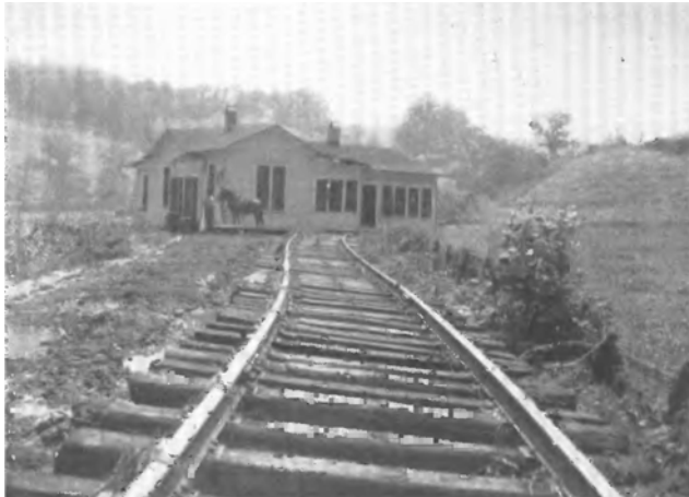
Figure 4: Residence near Heaters with its four occupants inside was washed one mile down O'Brien Fork of Saltlick Creek and lodged on a displaced section of railroad track (Source: USGS WSP 1134-B)
