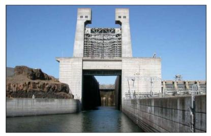
Figure G-2-7.—Overhead vertical lift gate.
