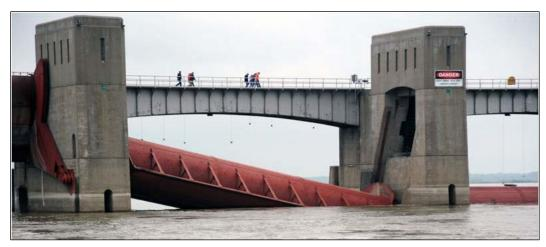
Figure G-2-18.—Damaged roller gate, Mississippi River Lock and Dam 25 (USACE 2011).
