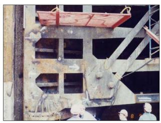
Figure G-2-13.—Fatigue cracking in girder flange at diagonal anchor plate, Markland Lock and Dam (USACE 2010b).
