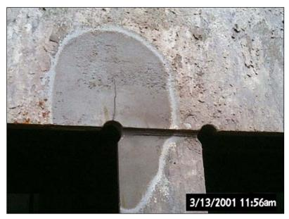
Figure G-2-17.—Fatigue cracking in the tension tie, vertical lift gate, John Day Locks and Dam (Hanson and Chambers 2001).
