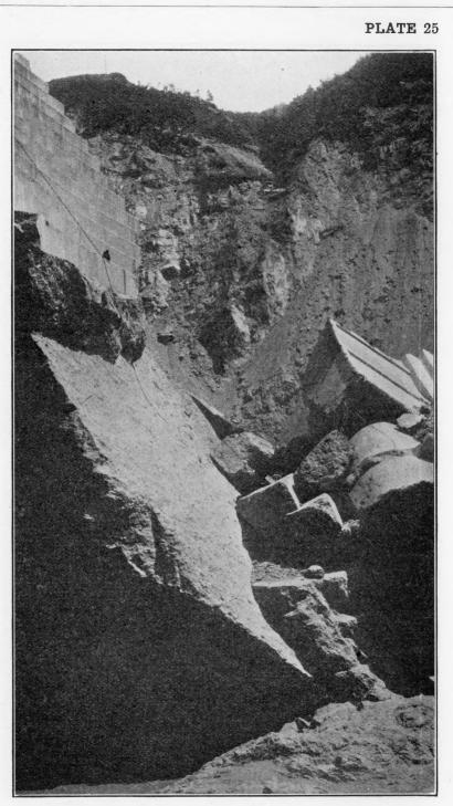
CONTACT PLANE BETWEEN CONCRETE AND FOUNDATION NEAR DOWNSTREAM TOE OF STANDING SECTION.
