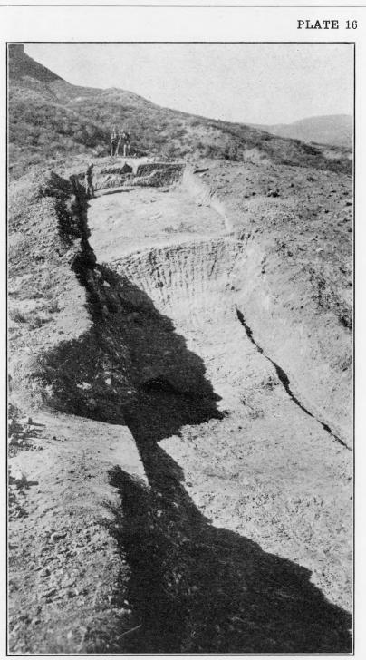
EXCAVATION FOR WING WALL SECTION.
