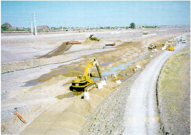
Figure 4. Slurry wall construction at toe of shoreline CSA
