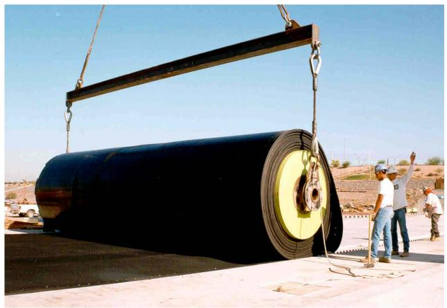
Figure 5. Rubber bladder being positioned on dam foundation
