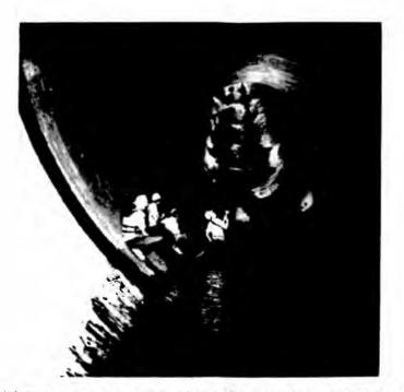
a. View looking upstream across flooded hole at cavitation damage in the vertical bend. Note that the tunnel liner has been removed well above the springline August 1983.
