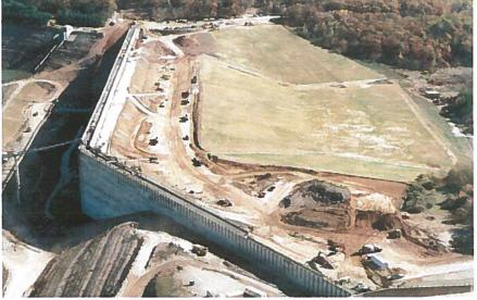
Overview of New RCC Dam With Regraded Embankment Against Downstream Face of the Dam
