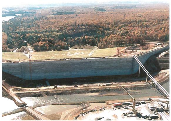
Looking at Upstream Face of New RCC Dam During Construction, September 1998
