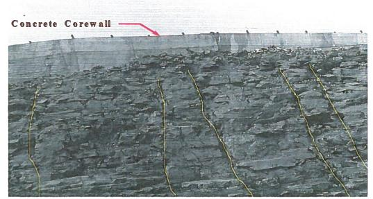
**Construction Photo of Concrete Core Wall on Fractured Rock Foundation**
