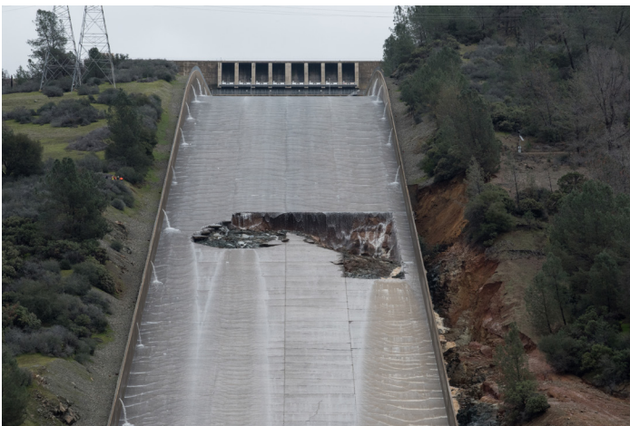
Figure 1: Oroville Dam Primary Spillway after Initial Failure (Ref. California Department of Water Resources)
