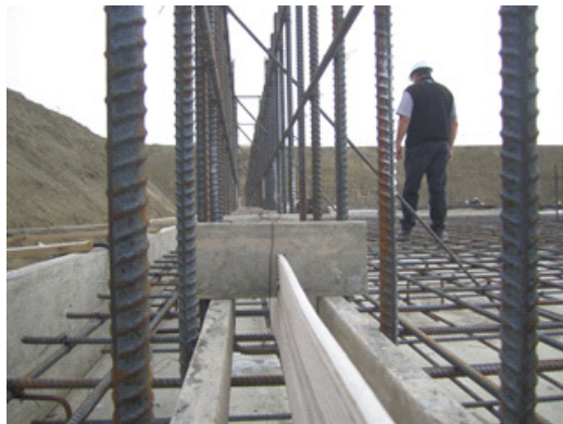
Figure 9: Properly Securing Waterstop (Ref. Sika Greenstreak)
