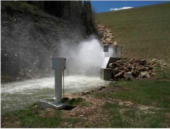
Photo 1: Releasing 300 ft 3 /sec through a Low Level Outlet at Dam in Utah
