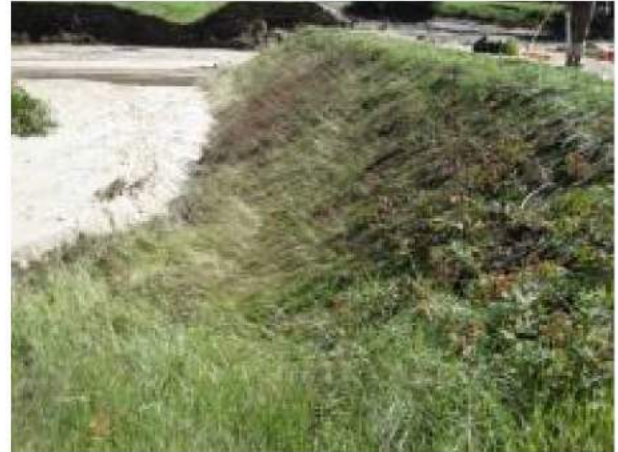
Photo 6: Downstream slope of Sunset Lake Dam after overtopping looking from left abutment.
