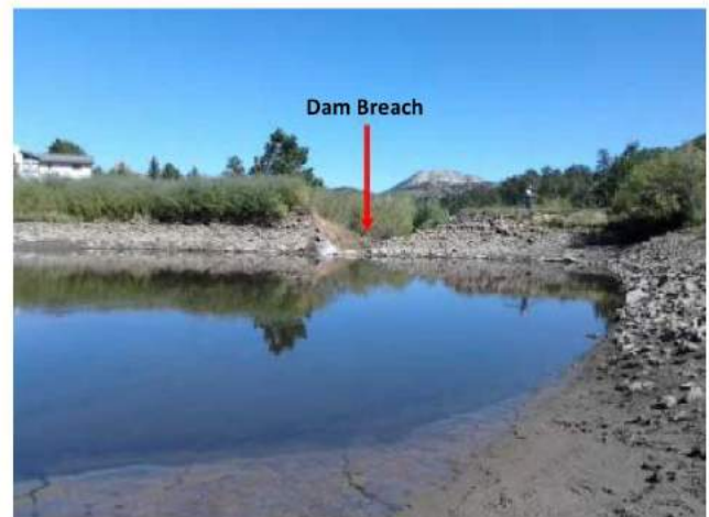
Photo 12: CH2 Dam post-failure looking downstream from reservoir. Note heavy vegetation on dam crest.
