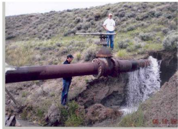
Photo 6. Damage Incurred to Outlet Conduit during Operation
