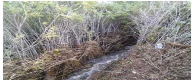
Photo 16: 2-foot-wide notch formed in CH1 Dam spillway.
