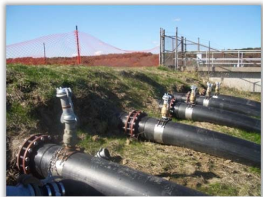
FIGURE 4 - VALVES INSTALLED ON A PIPE
