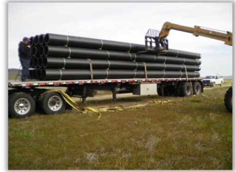
FIGURE 7 - HDPE PIPE BEING UNLOADED
