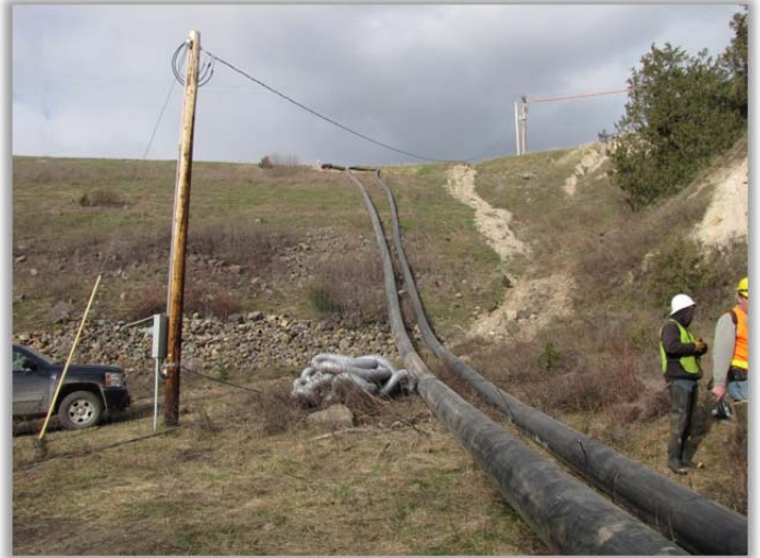
FIGURE 24 – PUMP DISCHARGE LINE
