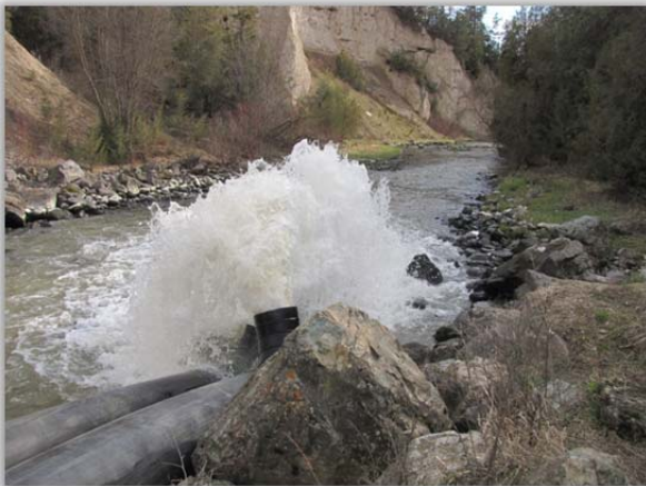
FIGURE 3 – A 90 BEND IS DIRECTED UP ON THE OUTLET PIPE TO DISSIPATE ENGERGY
