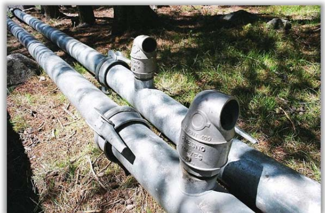
FIGURE 15 – AIR VALVES
