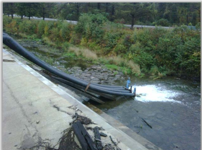
FIGURE 9 - OUTLET OF SIPHON WITH VALVES
