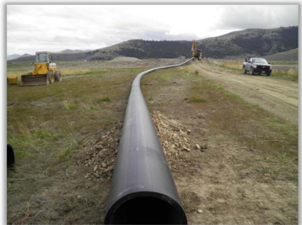
FIGURE 19 – HDPE BEFORE IT WAS PLACED
