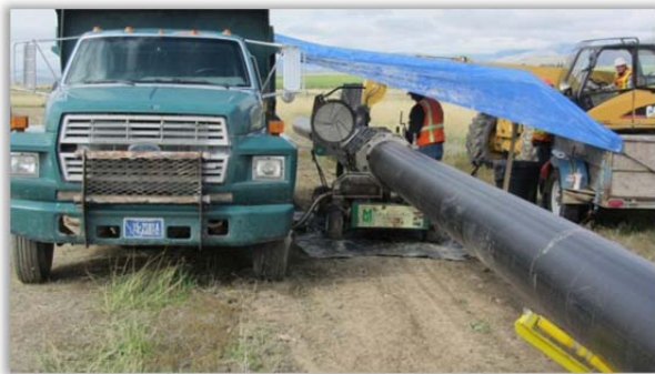
FIGURE 17 – FUSION OF HDPE PIPE
