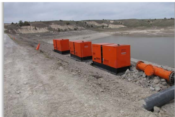
FIGURE 23 -DIESEL GENERATORS
