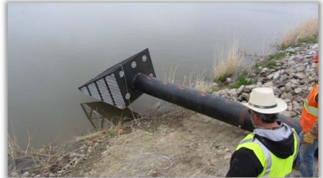
FIGURE 8 - INLET SCREEN ON SIPHON INTAKE
