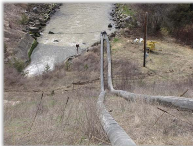
FIGURE 21 – DISCHARGE PIPE RUNNING DOWN CROW DAM EMBANKMENT
