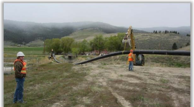
FIGURE 18 – PLACEMENT OF SIPHON PIPE
