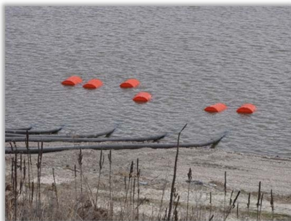
FIGURE 22 - SUBMERSIBLE PUMPS AND FLOATATION
