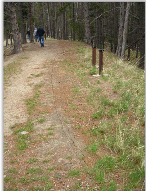
FIGURE 11 - CRACK IN DAM EMBANKMENT
