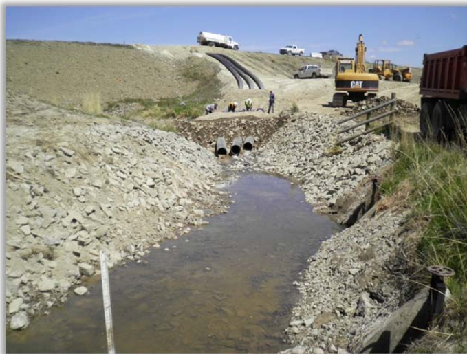
FIGURE 20 – BACKFILL BEING INSTALLED OVER OUTLET PIPE.
